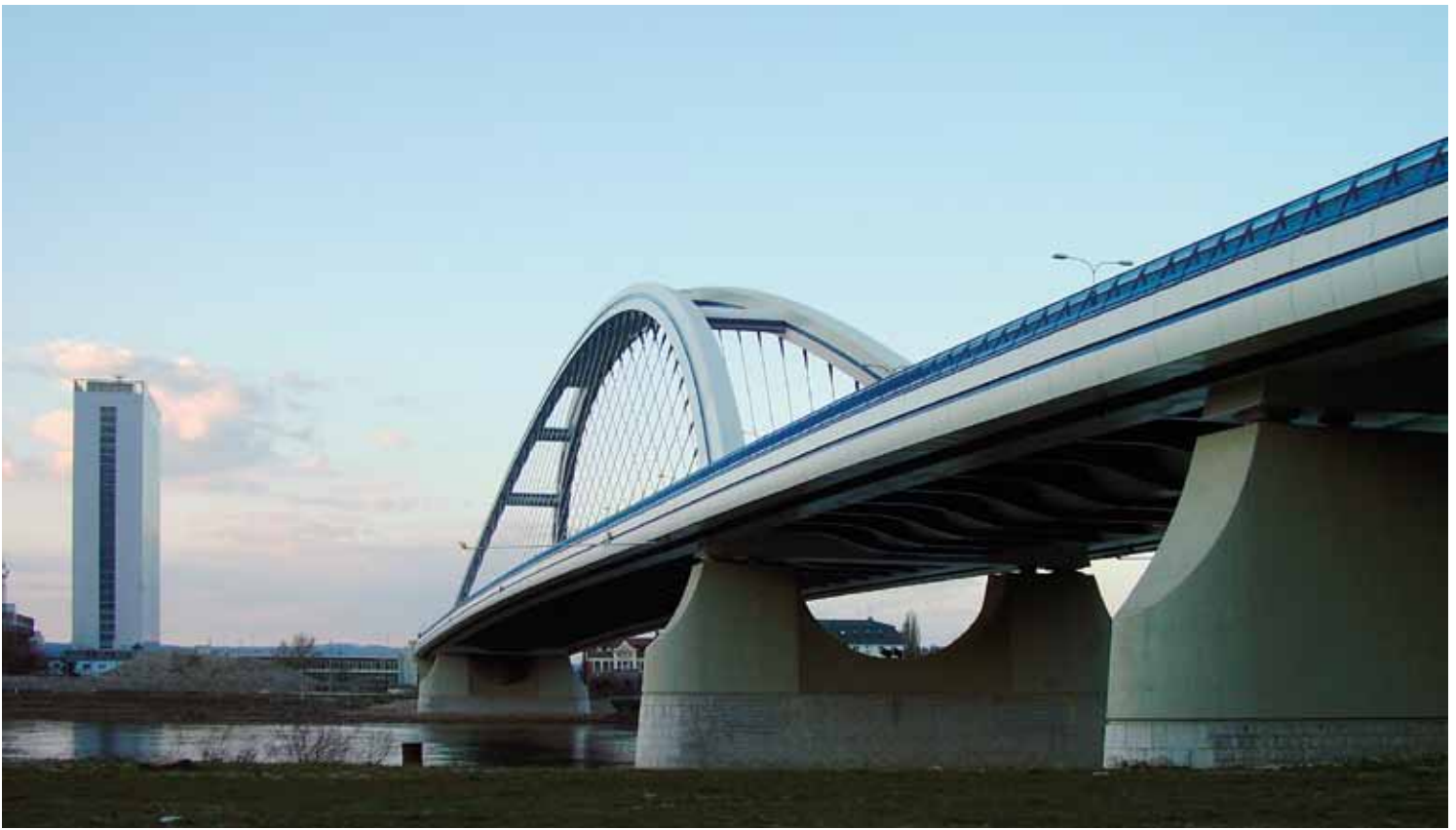
The first large structure in Slovakia designed according to Slovak national standards and ENV Eurocodes was the bridge Apollo over the river Danube in Bratislava.
